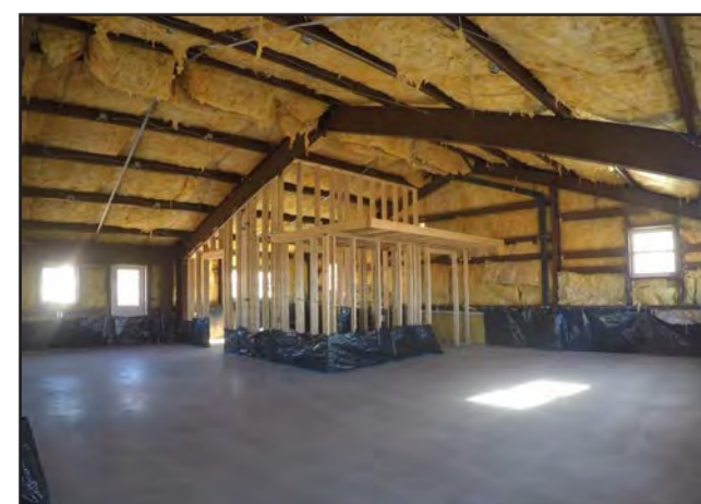
Top floor in preparation for concrete floor stain
