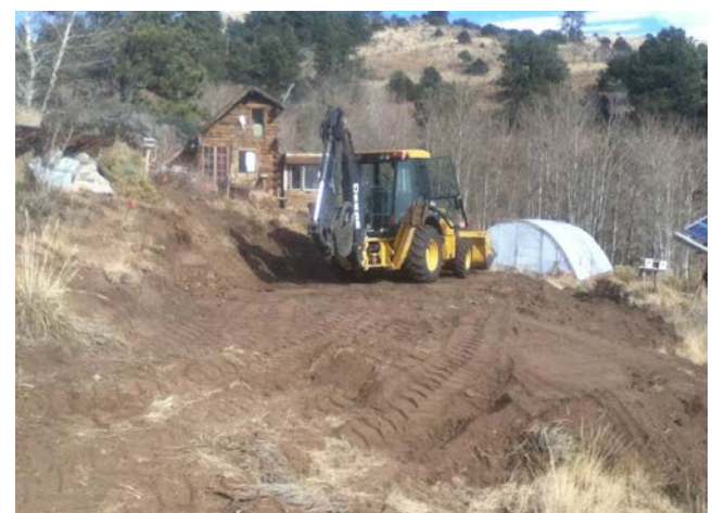
Clearing the foundation for the new greenhouse, November 2013 (Photo by Benjamin Hoffman)
